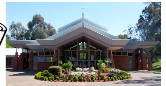
St Michael's Church Tyrrell Cct Kaleen
